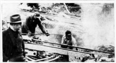
Toe hole drilling with Kennametal PX Rock Bits.
